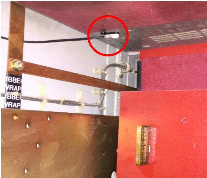
Fig. 7 Point Sensor Mounting Detail
