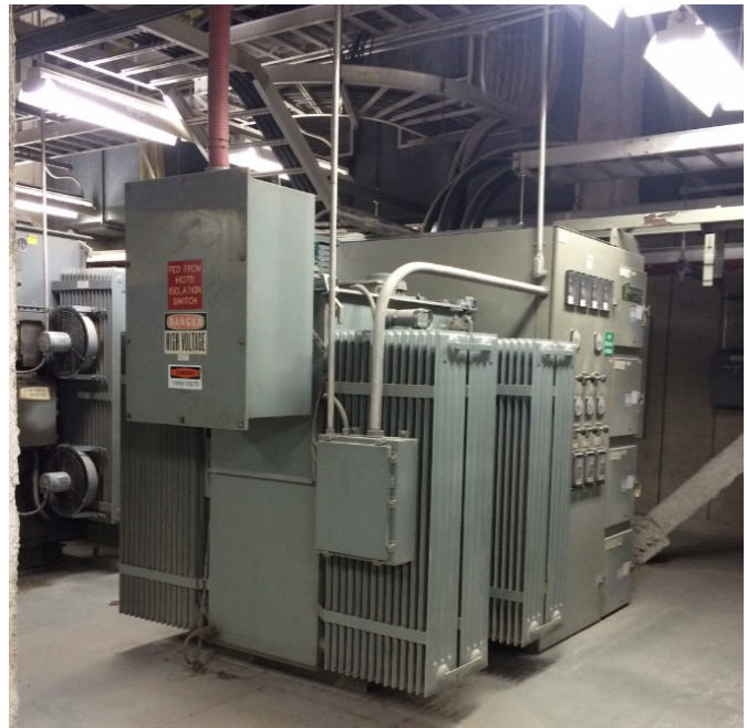
Fig. 1 Close-Coupled Transformer and Switchgear
