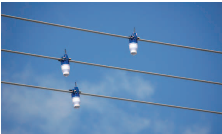
These fault indicators communicate fault information via a wireless network.
