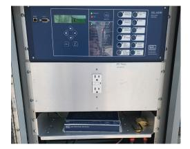
Figure 7—SEL-FR12 installed in the SEL-651R recloser control cabinet.
