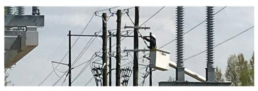
Figure 9—A line worker installs an SEL-FT50 outside the Northside substation on the overhead section of the feeder.
