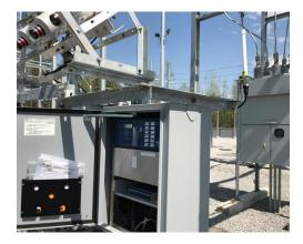
Figure 8—Omnidirectional antenna connected to SEL-FR12 to communicate with SEL-FT50 transmitters.
