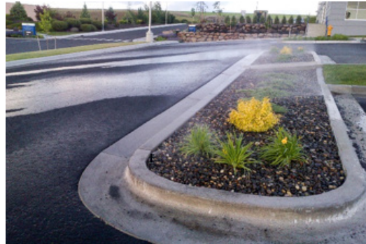
Figure 2—Water Runoff on SEL Zocholl Parking Lot
