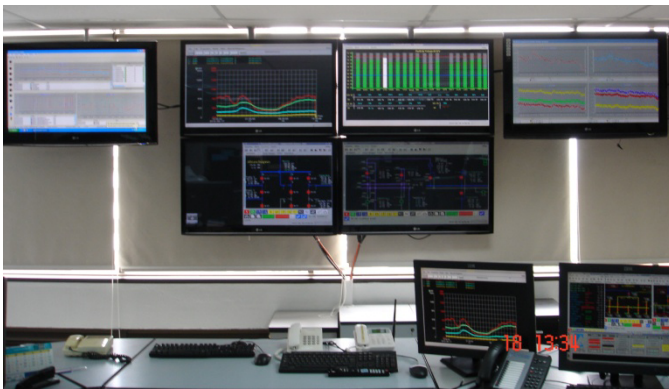
Fig. 5. Synchronphasor data complement traditional SCADA
