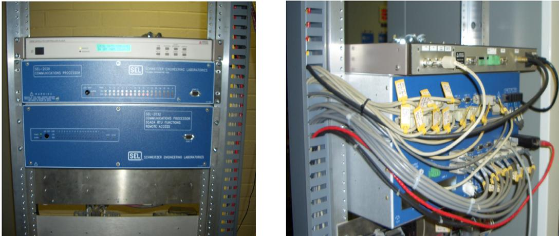
Figure 6 Satellite Clock, Communications Processors, and IED Data Communications
