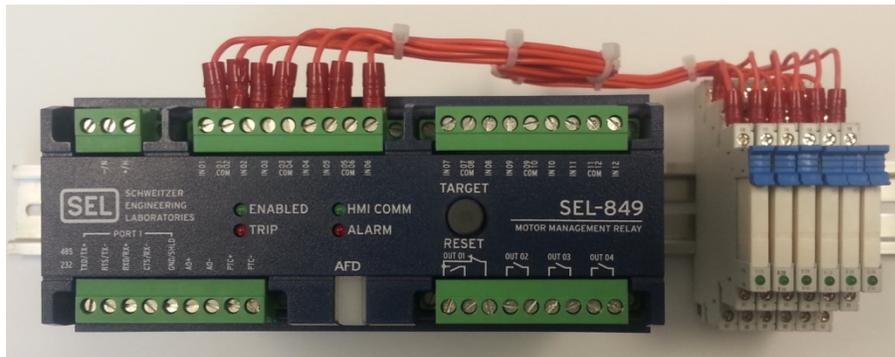
Figure 3 SEL-849 With Interposing Relays
