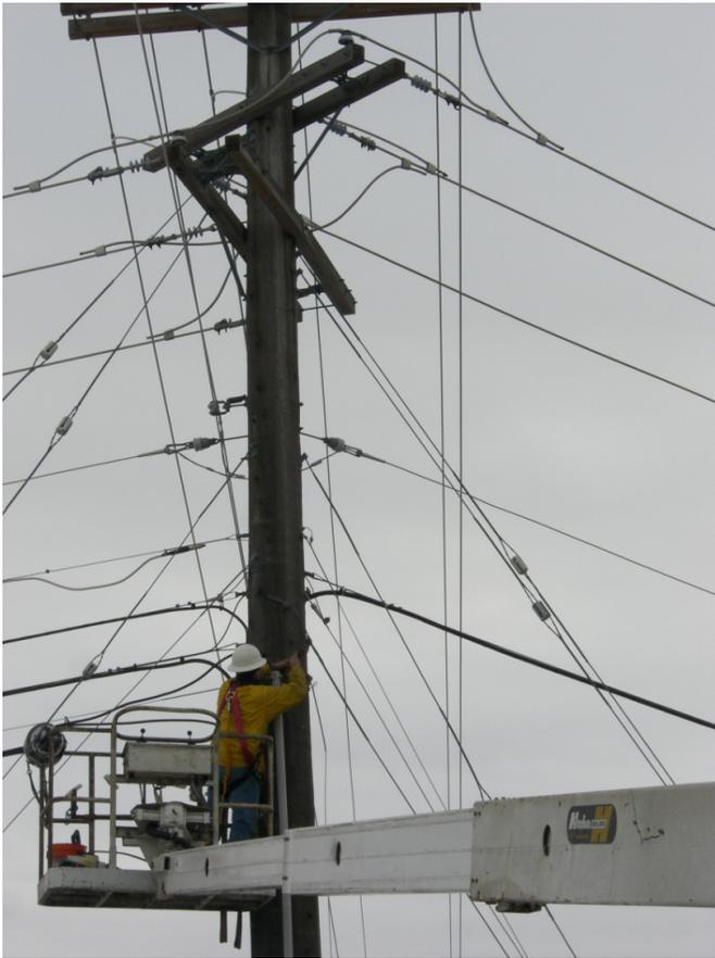
Fig. 5. Dual feed and underground transition on distribution feeder.
