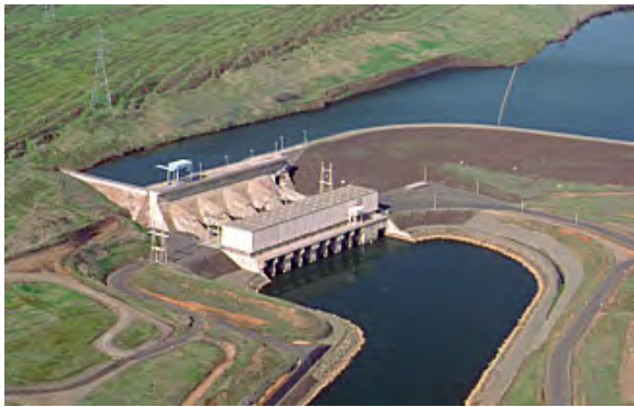
Fig. 2. Thermalito Power Plant
