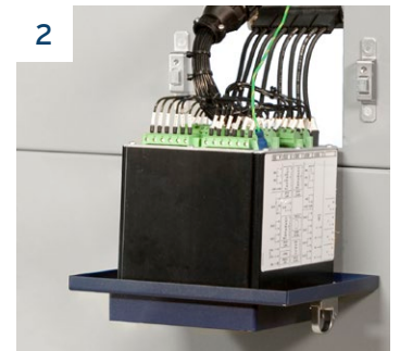
2 Hinge meter down.
