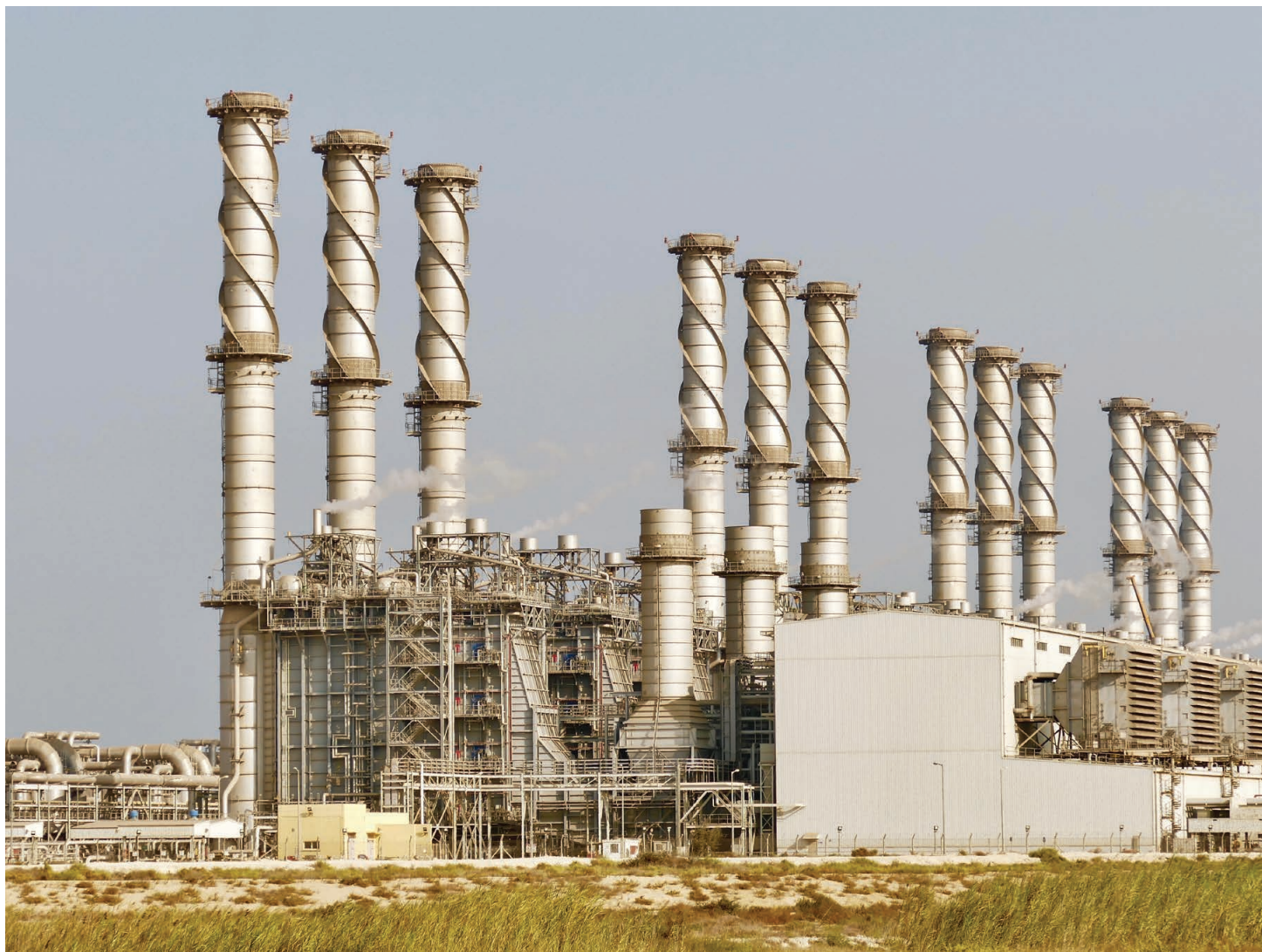
▲ JUBAIL WATER AND POWER COMPANY
