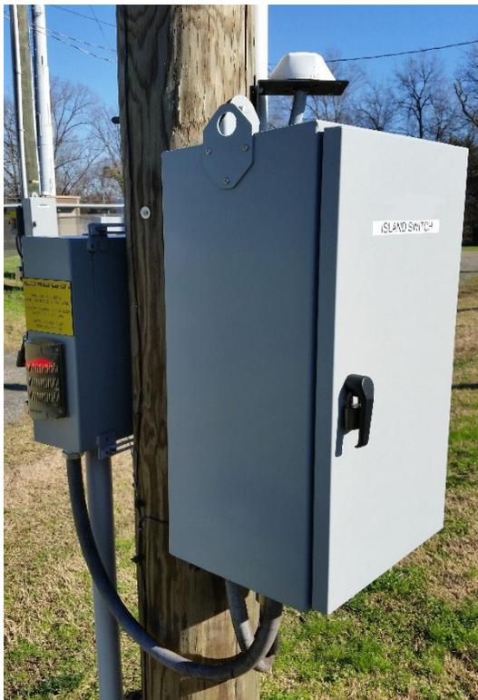
Fig. 16. ISO Switch Control With Signal Light
