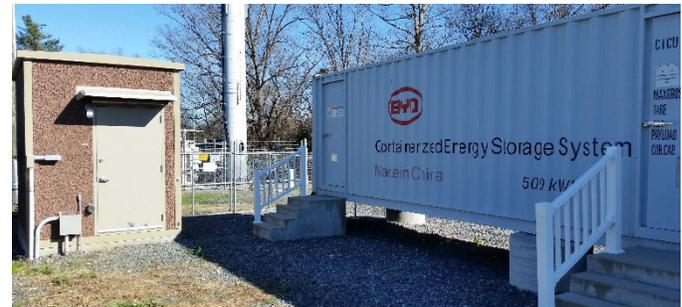
Fig. 14. Control House Exterior and BESS
