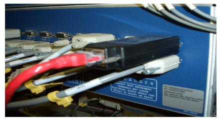
Figure 7 Serial-to-Ethernet Converter on the Communications Processor for SCADA Access
