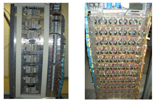
Figure 3 Using the Communications Processor's Multifunction Control Capabilities Eliminated all of the PLC Inputs, Control Outputs, and Interposing Relays Shown in These Two Photos
