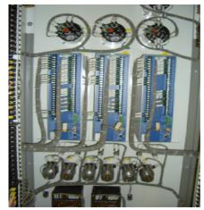
Figure 2 Utilizing Relay I/O to Eliminate PLC I/O
