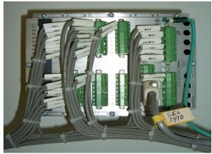
Figure 4 Transformer Monitor Wire Terminations to I/O Processor Analog and I/O Cards and Serial Connection to the Communications Processor
