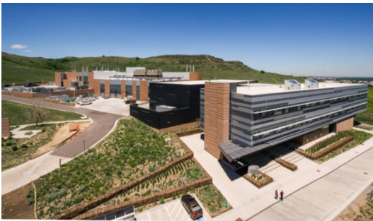
Figure 1—The NREL ESIF (photo courtesy of Dennis Schroeder)
