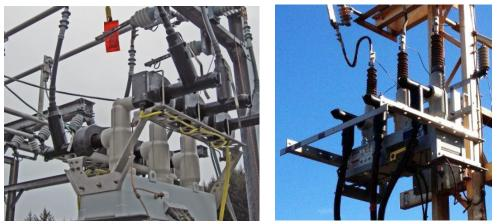
Figure 11 Elbow-Connected G&W Viper Reclosers
