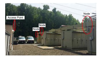
Fig. 3. Access Point and Communications Nodes in a Substation Yard
