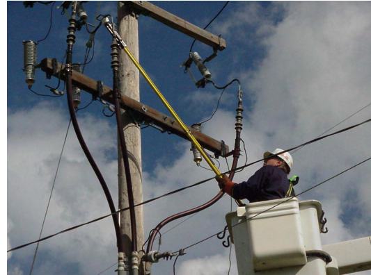
Figure 1—SEL ERL fault indicators lead utility service personnel to fault locations so they can quickly restore service to customers.
