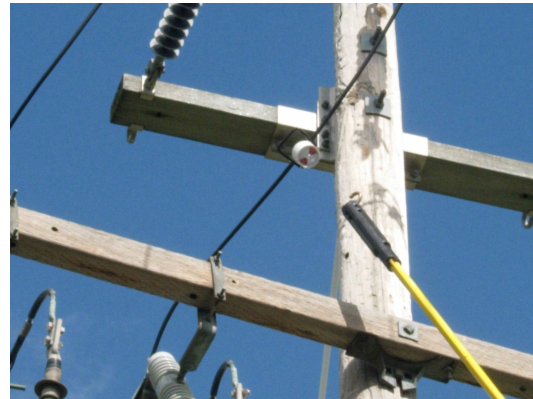
Figure 5—FCI installation orders became part of the company's work management process.
