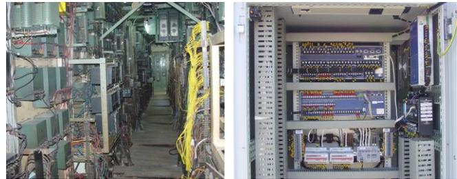
Fig. 4. Old and New Relay Panels
