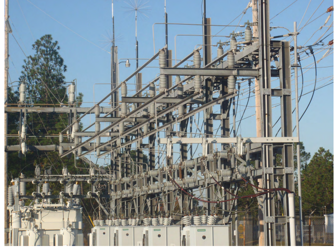
Fig. 3. Main and Transfer Bus Arrangement
