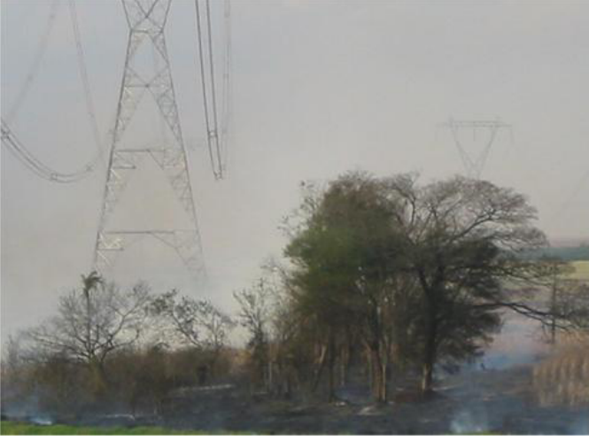
Fig. 7. Fire damage visible at fault location
