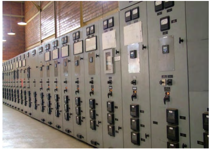
Fig. 10. Students created settings for digital relays to replace electromechanical relays on feeders in the WSU steam plant.
