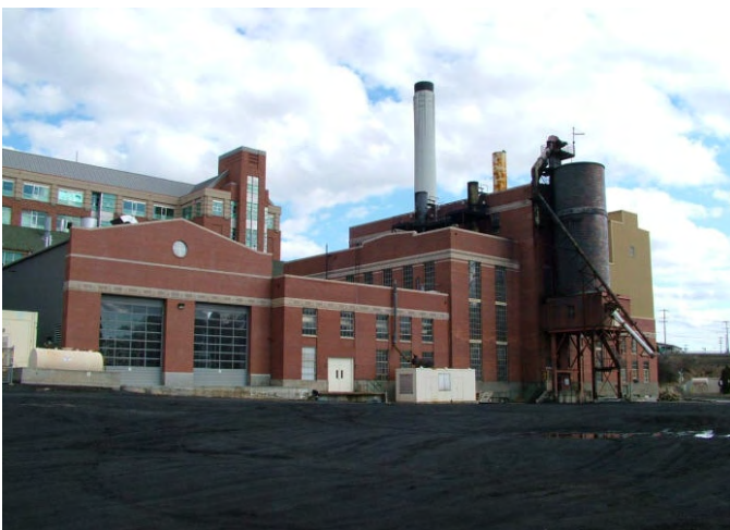
Fig. 9. WSU steam plant.
