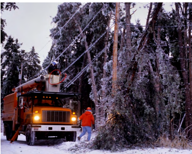
Fig. 3. Electrical line workers respond in harsh conditions.
