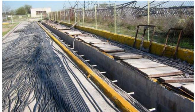
Fig. 1. Copper cable replacement
