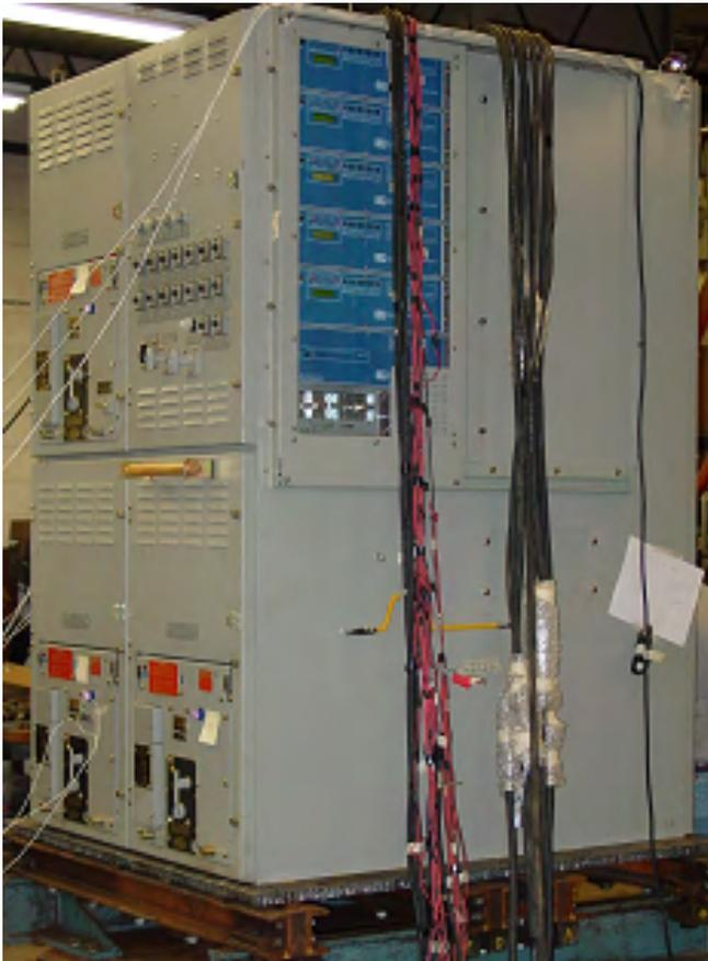
Fig. 4. Partial 4160 V Switchboard With MFMD
