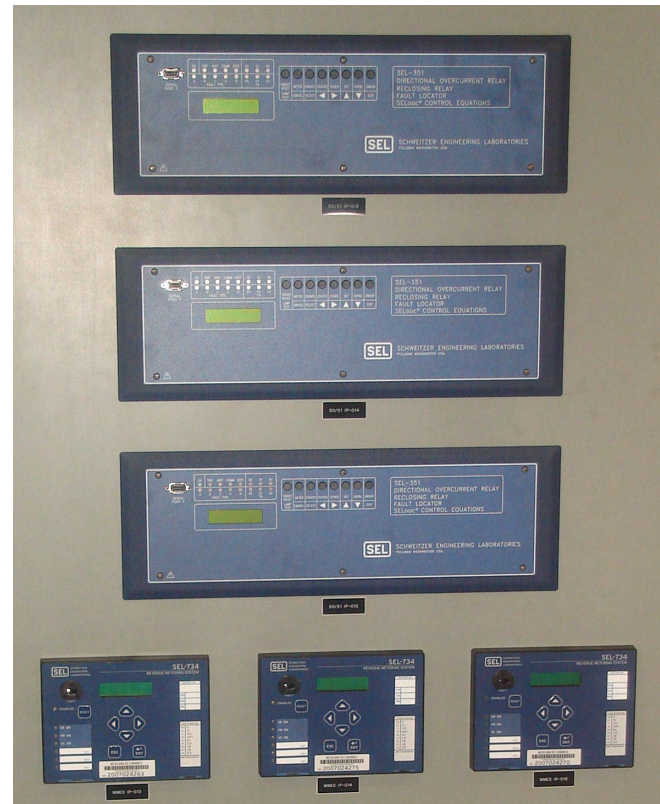
Figure 3.4 SEL protection, control and metering panel for three feeders. Three SEL-351 relays replace nine phase relays, three ground relays, three reclosing relays, and many auxiliary relays.
