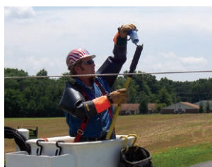
Install the Overhead AutoRANGER with a single hot stick.
