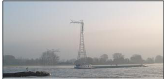
Fig. 45. Tower and feeder damage from impact of large helicopter (photo source unknown).
