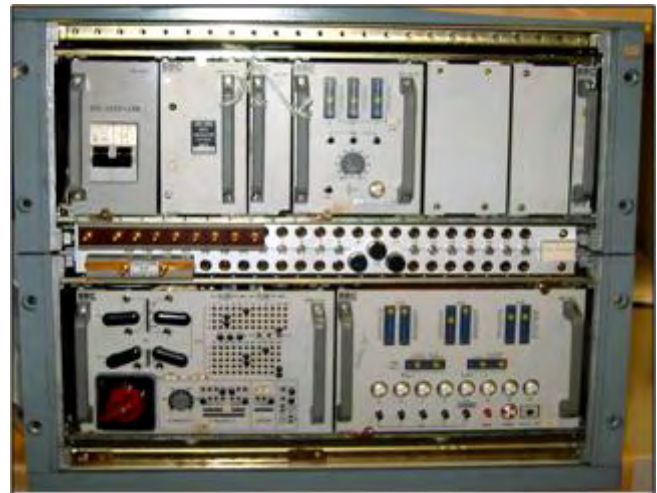
Fig. 31. Second generation (solid state) protection relay
