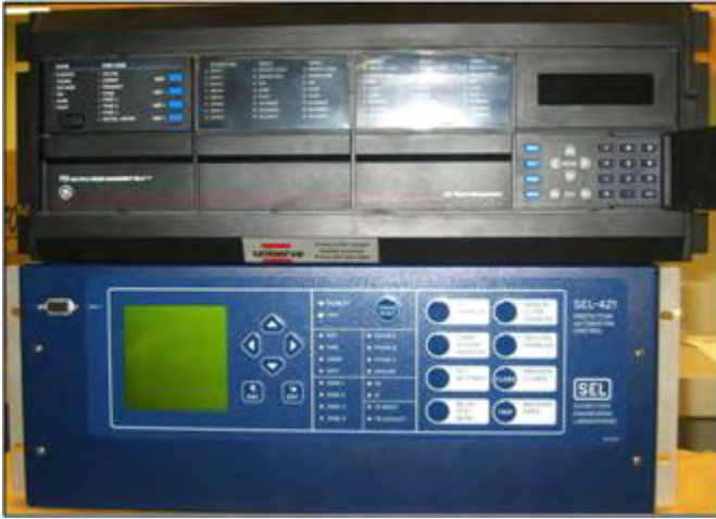
Fig. 32. Third generation (numerical) protection relay.
