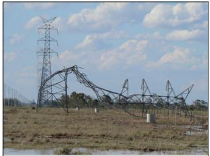
Fig. 46. One of seven collapsed towers resulting from a storm cell—OPGW was stretched but still operational
