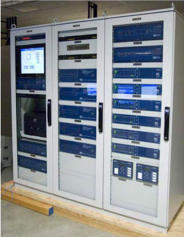
Fig. 9. Saudi Aramco Shaybah Oil Refinery power management LPS
