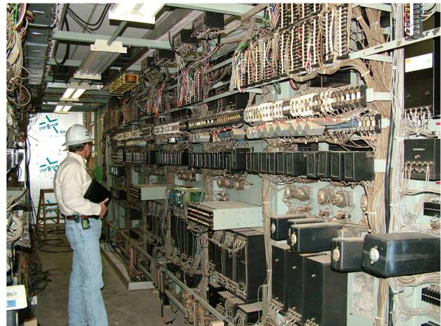
Fig. 4. Electromechanical relay panel with rear-panel wiring. This photo is courtesy of Oncor.
