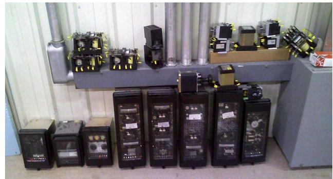
Fig. 2. Electromechanical distance scheme components.
