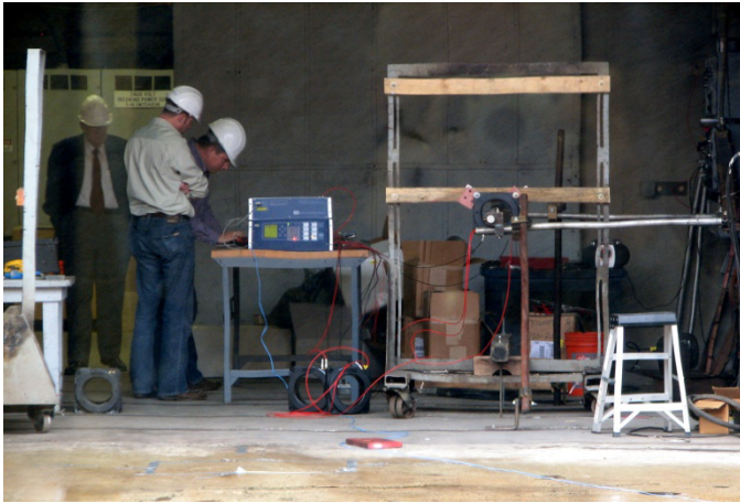
Fig. 25. High Primary Current Test Cell With Test CTs, High-Impedance Bus Differential Relay, and Monitoring Relay
