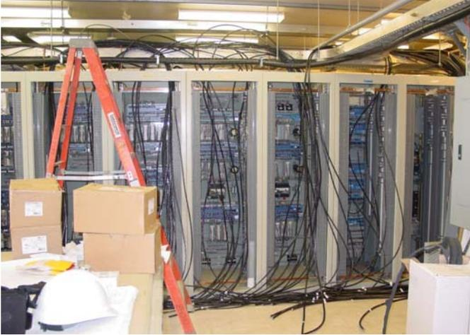
Fig. 8. Portage la Prairie South Protection and Control Panels During Installation
