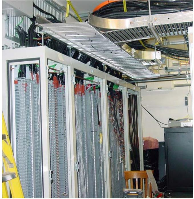
Fig. 9. Termination Cubicle With Station Simulator (in Black)
