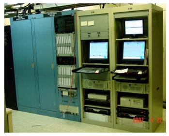
Fig. 5. Standard Manitoba Hydro RTU and HMI Installation
