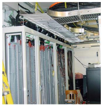
Fig. 9. Termination Cubicle With Station Simulator (in Black)
