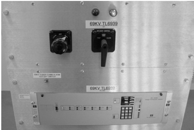
Figure 17 SDG&E Differential Relay 1
