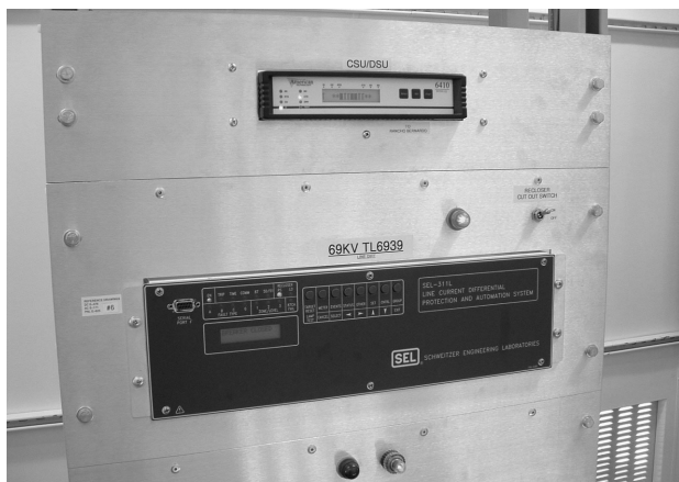
Figure 18 SDG&E Differential Relay 2 Front View
