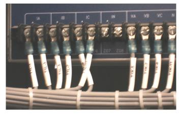
Fig. 20. CT Polarity Wiring Problem Found and Fixed
