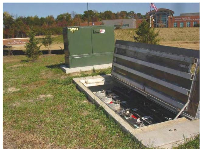
Fig. 6. High-speed fault-clearing system installed at Cyber Park
