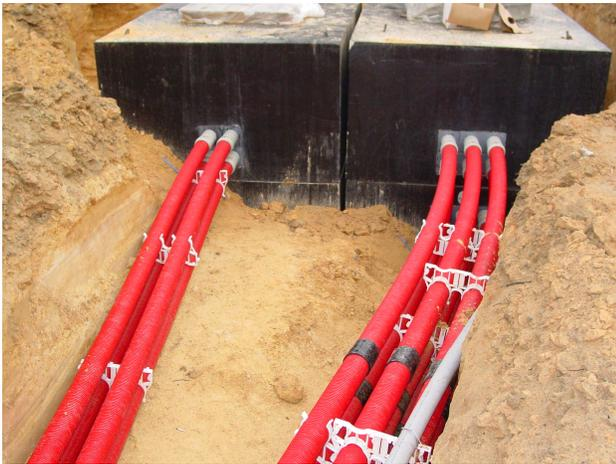
Fig. 2. Direct-buried conduit for fiber link and high-voltage cables
