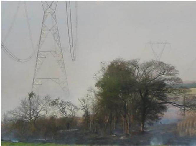
Fig. 7. Fire damage visible at fault location
