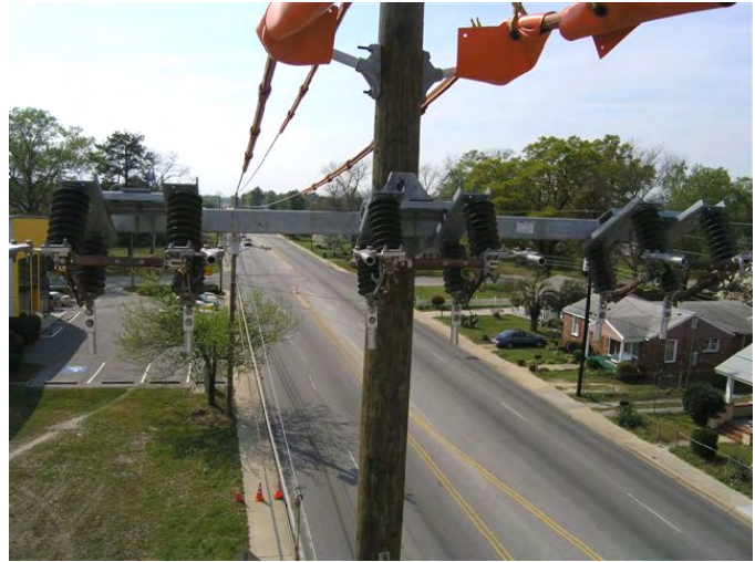
Fig. 3. Bypass arrangement used on another recloser installation of the same type as mentioned in this paper
