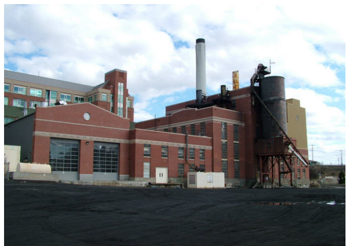
Fig. 7. WSU steam plant
