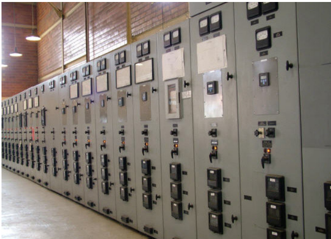
Fig. 8. Students created settings for digital relays to replace electromechanical relays on feeders in WSU steam plant
