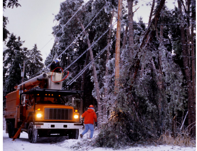
Fig. 3. Electrical line workers respond in harsh conditions
