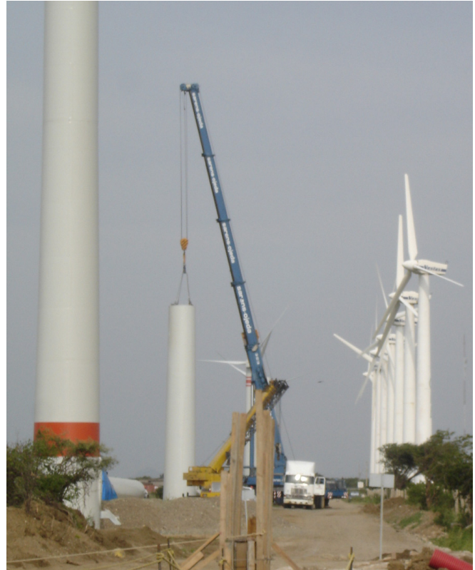
Fig. 14. Construction of Wind Farm La Venta II
