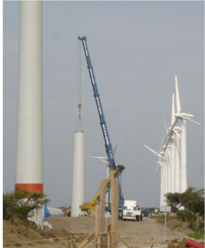
Fig. 16. Construction of the wind farm
