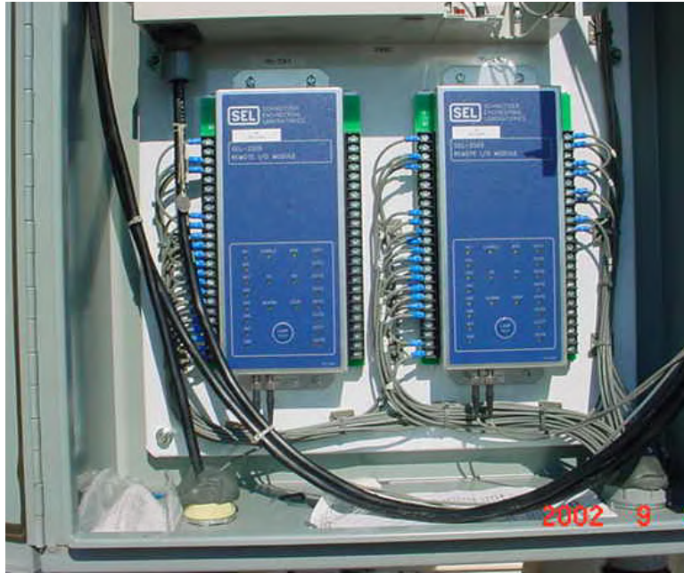
Figure 3 The I/O device on the right provides open and close commands for the MODs. It also provides the 43LR, 52a, and 52b status to the DCS. The I/O device on the left provides inputs into the DCS for the individual power circuit breakers. Note the extra fiber-optic cable, which allowed terminations to be completed in a mobile van and provided additional cable for when the power circuit breaker is replaced.
