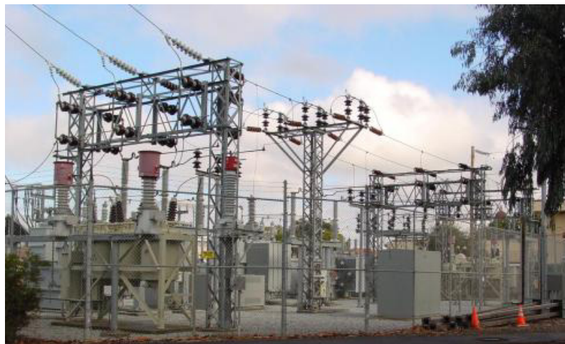
Figure 7 Palou Substation—Obsolete Oil Circuit Breaker (OCB) on Left
