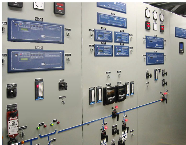
Figure 9 Palou Substation—New Protection and Control Panels
