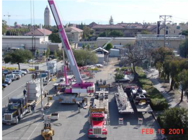
Figure 6 33 MVA Transformer During Installation
