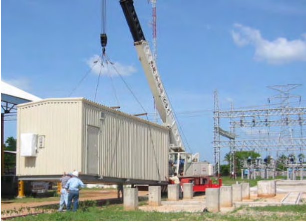
Fig. 5. New KLV Control House
