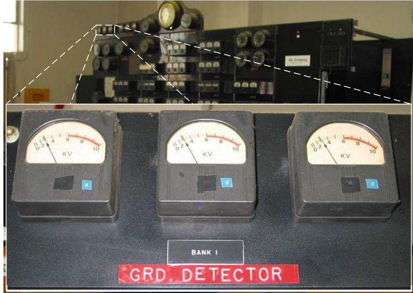
**Figure 4** Existing Ground Fault Detection System Consists of Phase Voltage Meters
