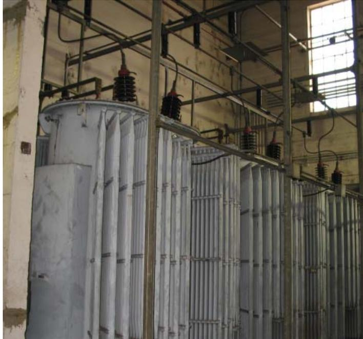
**Figure 6** Power Transformer Bay and Overhead Bus Work Are Compact
