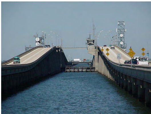
Figure 2—A new electrical system was needed to power drawbridge operation, cell phone towers, toll facilities, and a series of variable-message warning signs to be installed along the, oftentimes fog-enshrouded, causeway.
