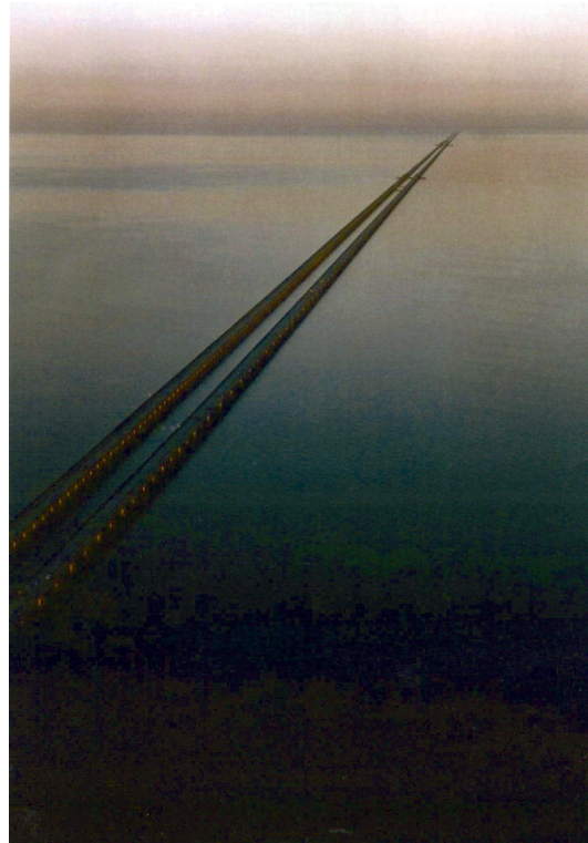
Figure 1—Photographed at dusk the Lake Pontchartrain Causeway originally constructed in 1956 was expanded to two-twin lane spans in 1969. The 24-mile long causeway is a vital link between New Orleans and the communities to the north and is the primary hurricane evacuation route for coastal areas.
