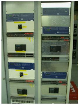
Figure 3—The Iroquios Falls mill protection system utilizes GPS-synchronized time and the Ethernet LAN to communicate records, data, and Sequential Events Recorder files from the SEL relays. This exact information is used for reconstruction and analysis of events.
