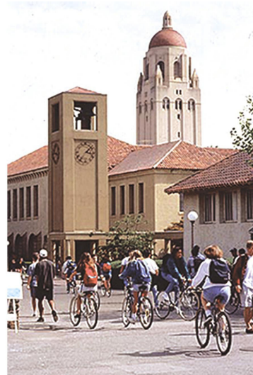
Figure 1—Located beside Palo Alto in the San Francisco Bay area, Stanford University is more than a medium-size city unto itself; it is a highly developed and complex campus. The ever-mounting electric energy needs include providing for a vigorous real estate development plan. When the plan is fully implemented, the campus will house thousands of buildings and an even higher population of users who will be highly dependent on reliable electric power.
