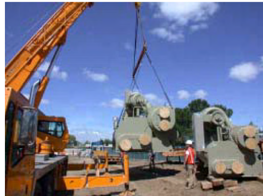
Chiller Unit Installation
