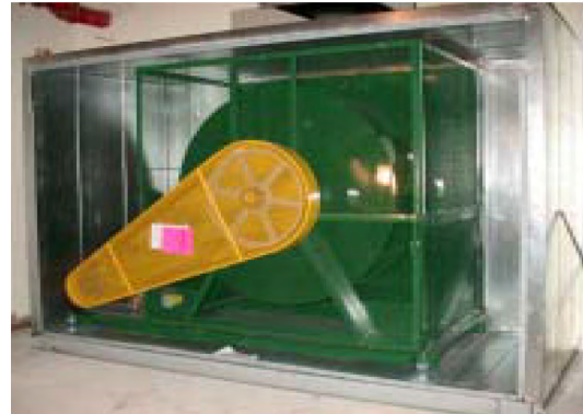
80,000-cfm Air Handling Unit
