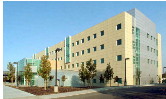
Figure 1—The TSF houses a total of 48,000 square feet of computer space with a projected load of 23 MW. The facility requires reliable electric power to ensure that the computations are not interrupted.
