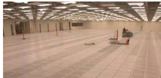
Figure 2—The computer room shown is 24,000 square feet of unencumbered space with a 48-inch raised floor. This room houses equipment capable of exceeding 100 tera-FLOPS at peak performance.
