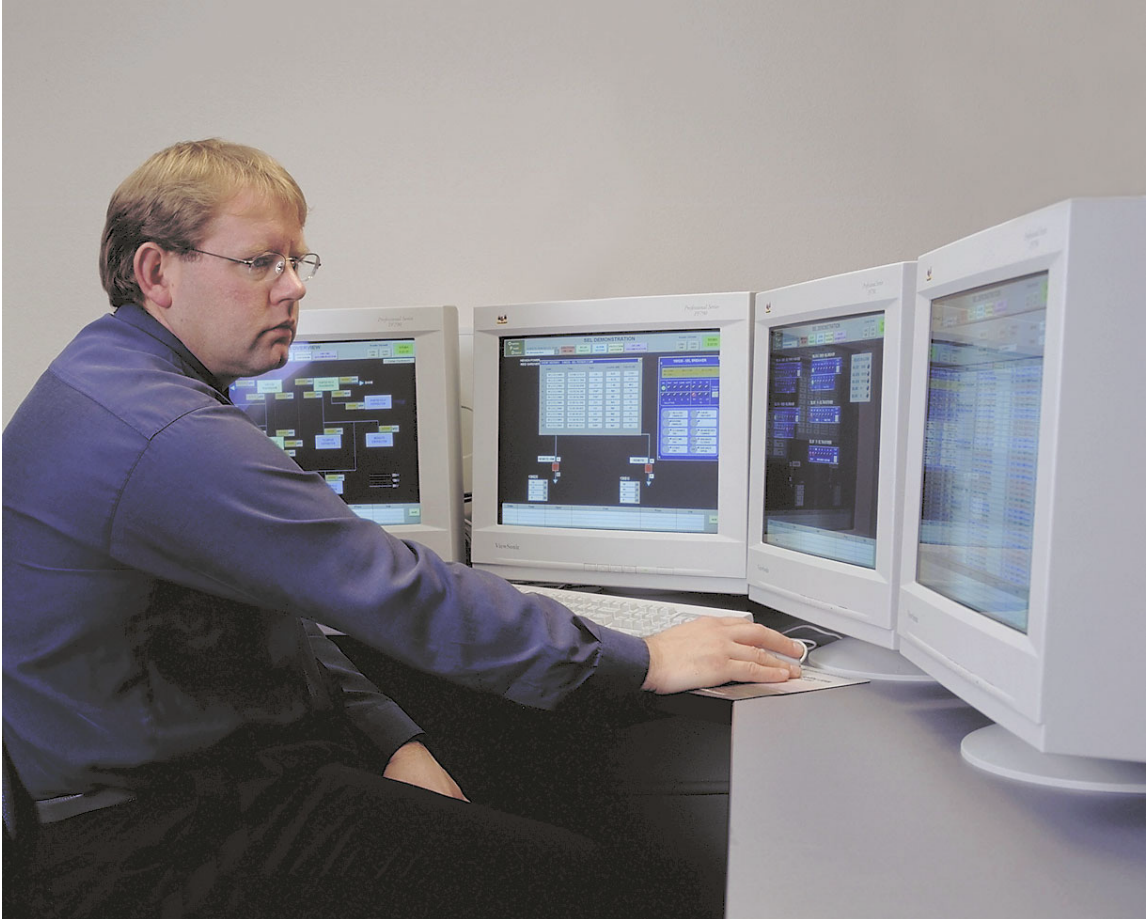
Figure 4 Four-Monitor Control Station
