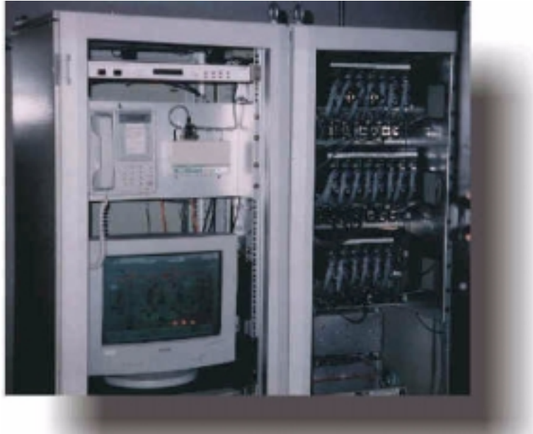
Figure 10: Programmable Logic Controller Right Cabinet, PC and Accessories Left Cabinet
