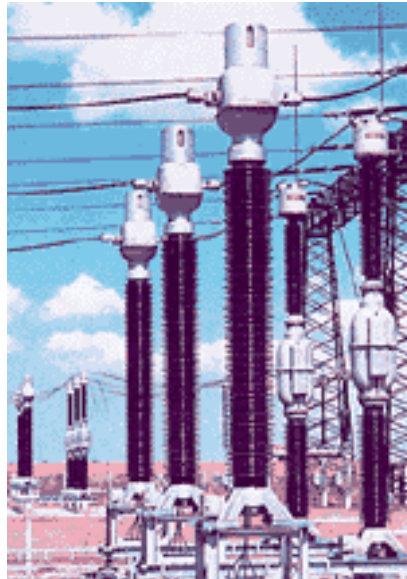
Figure 1: Instrument Transformers
