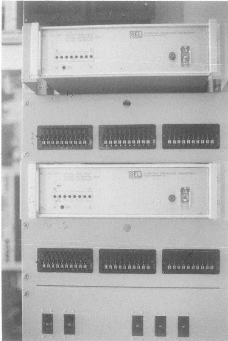
**Figure 21: New Capacitor Control and Protection Panel**
